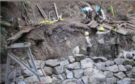
CCC remove the old bridge in preparation for the repair work.
