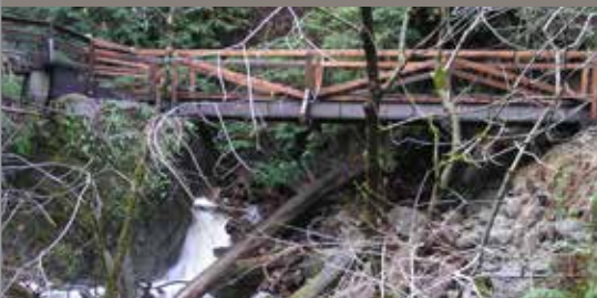
The newly rebuilt bridge spans Rattlesnake Creek.
