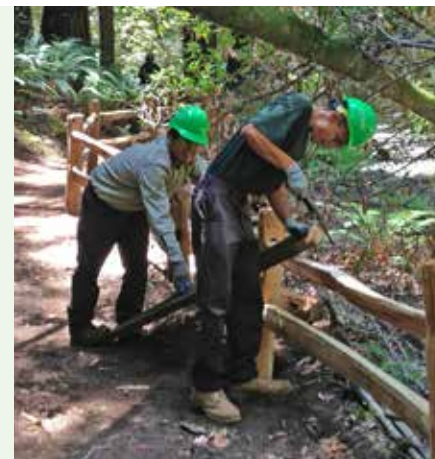
Crew members carefully replace sections of split rail fencing near fern Creek.
